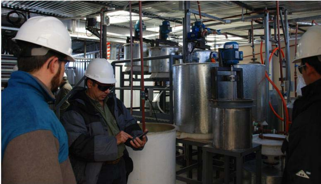
Process Development Facilities at Salar de Olaroz
